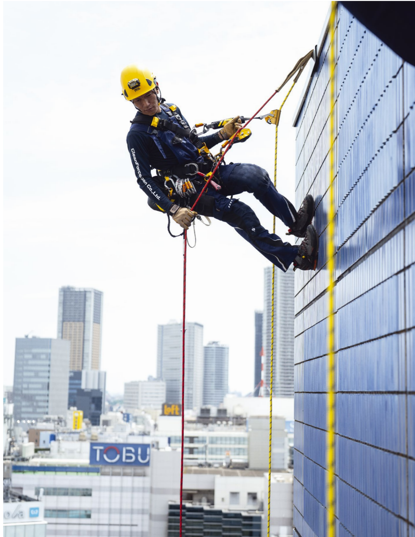
Rope access work at the Tokyo Metropolitan Theater © 2025 Petzl Distribution - Vuedici.org - Tokyo Metropolitan Theater - Clean Force Japan
